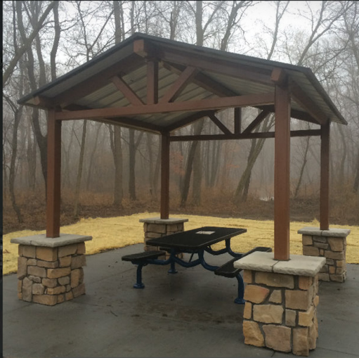
Rotary Club Shelter Dimensions: 12ft x 12 ft on Concrete slab: 20ft x 20ft
