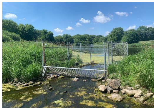
Figure 12. View of push trap during low water
