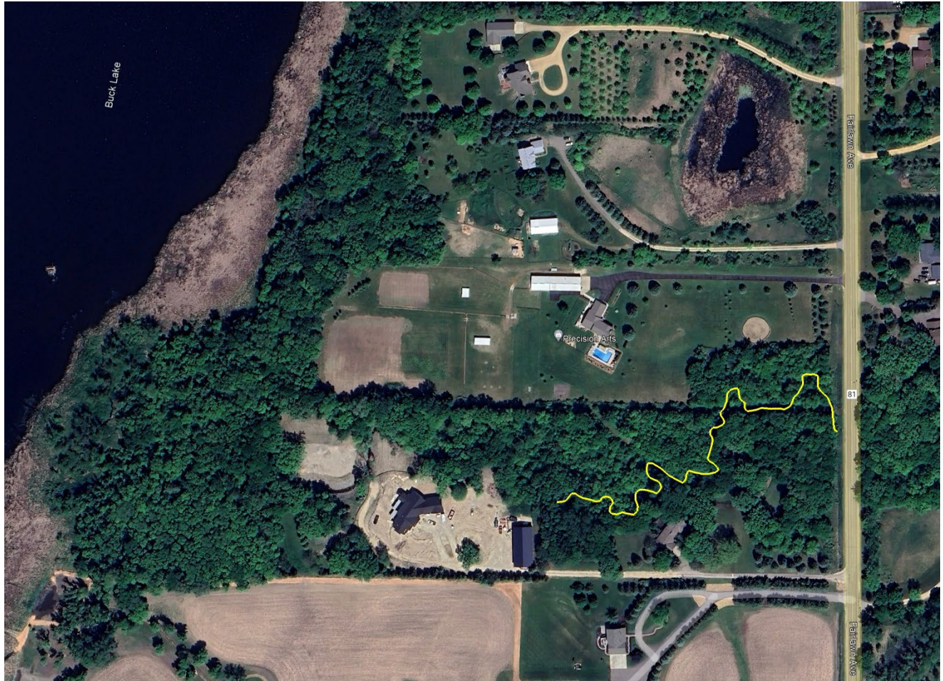
Figure 1. Location of proposed Buck Stream bank stabilization project (yellow line) west of Fairlawn Avenue.
