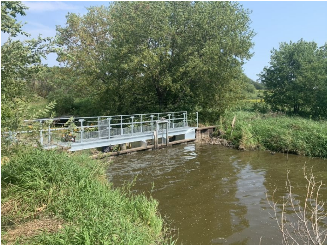
Figure 3. New walking deck over weir and fish barrier completed in 2020
