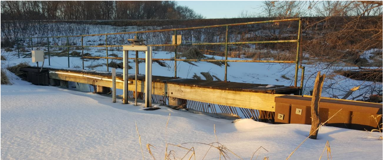
FIGURE 7 FERRIC CHLORIDE WEIR AND FISH BARRIER
