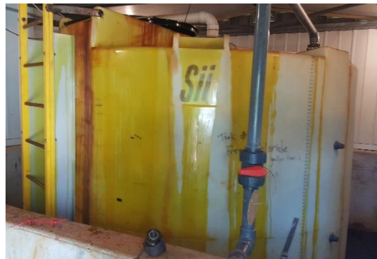
FIGURE 6 TANK OVERFILL
