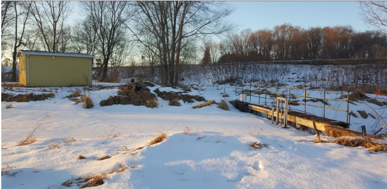
FIGURE 1 FERRIC CHLORIDE SHED AND WEIR
