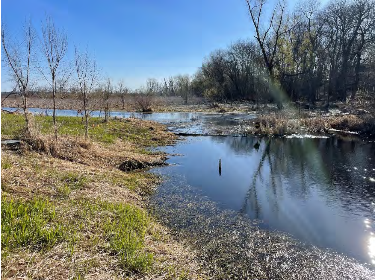
Figure 7: Water Flowing Untreated Over the Weir, With Tailwater Nearing Weir Level, Spring 2023.
