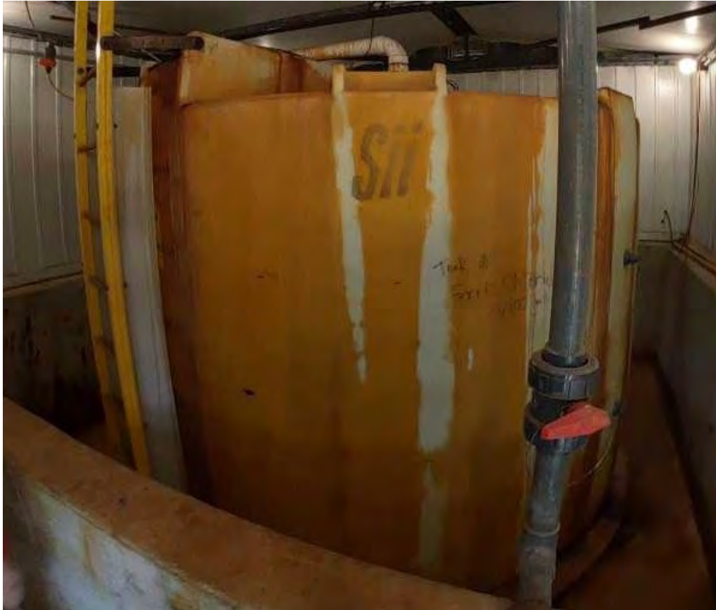
Figure 2: Existing Chemical Storage Tank.
