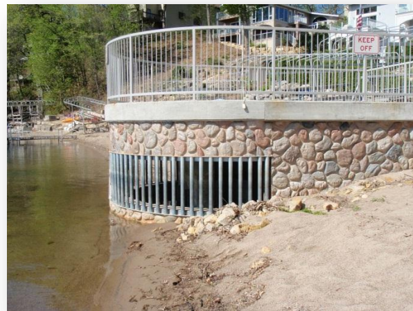
Prior Lake Outlet Structure
